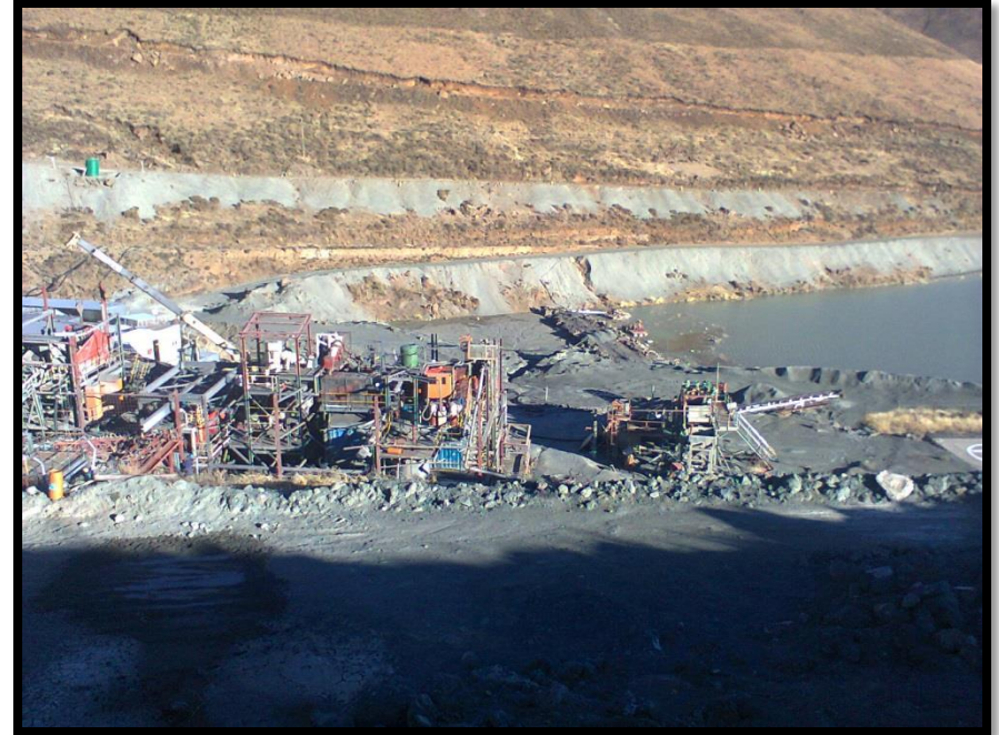
Pilot plant being dismantled
