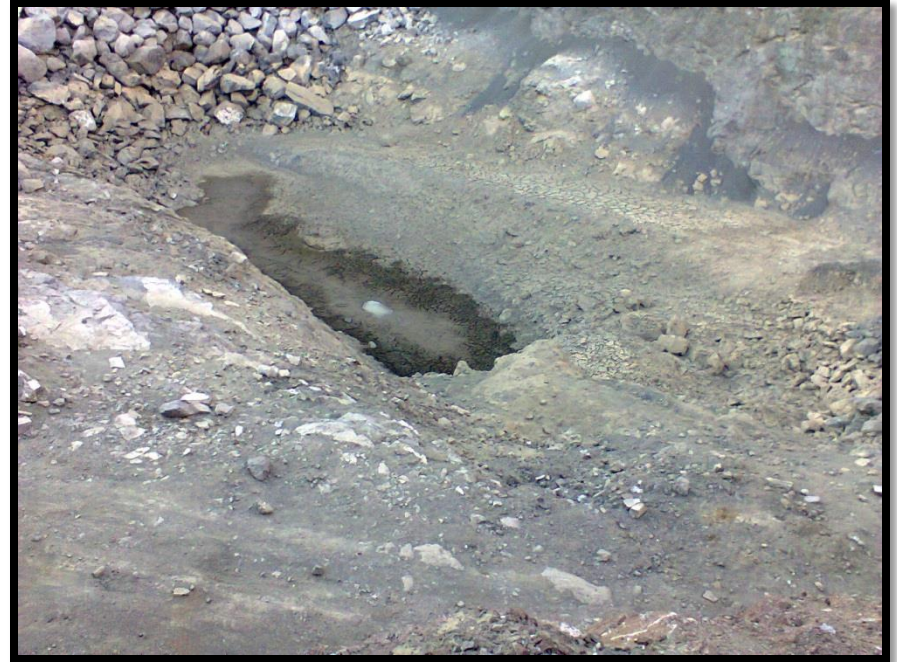
Satellite pit fully drained in preparation for deepening
