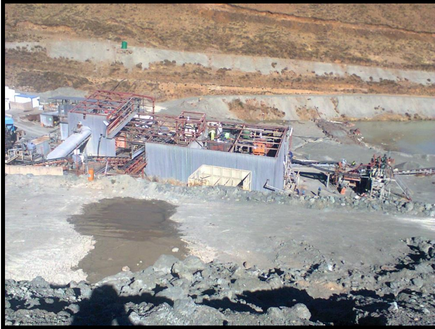
Pilot plant being dismantled
