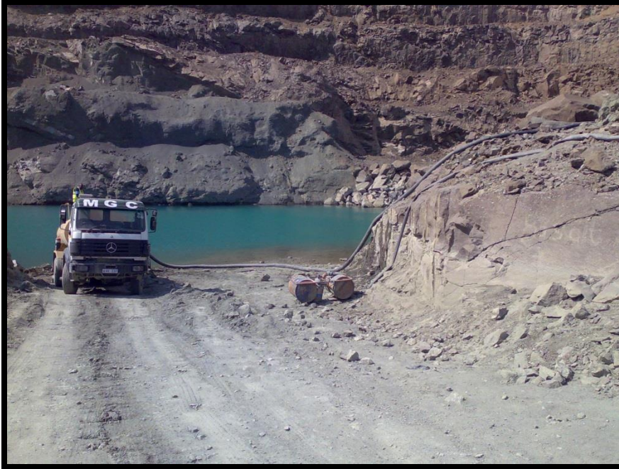
Satellite pit being drained
