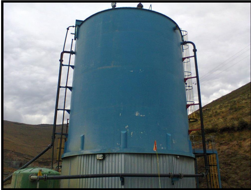
Thickener prior to being dismantled
