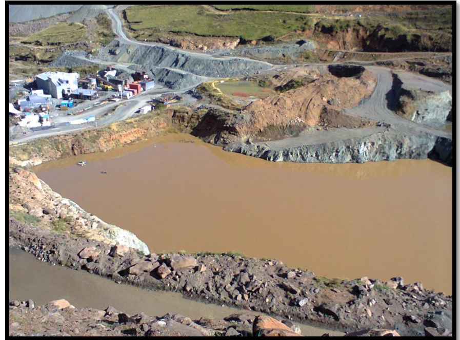
Main pit temporary water storage complete
