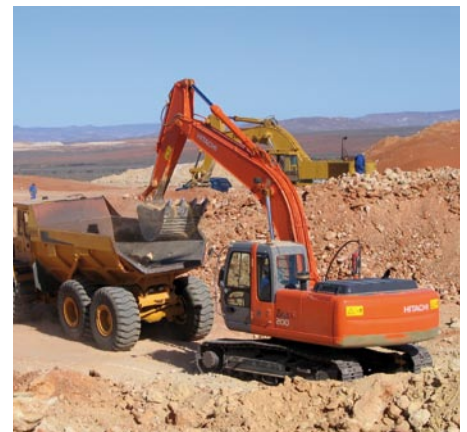
Overburden stripping, Bonte Koe Mine, South Africa
