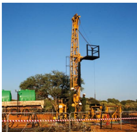
Core drilling, MK1, Tsabong
