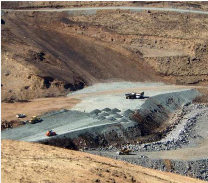
Toe of new slimes dam wall September 2014
