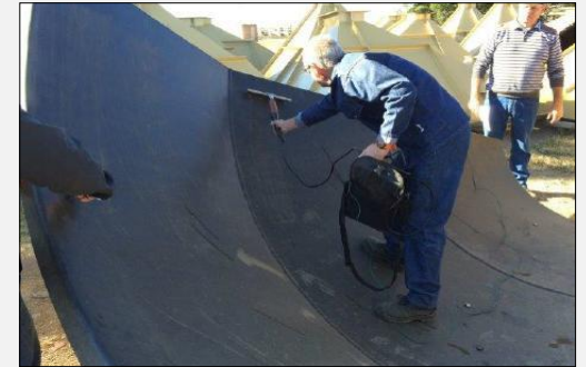
Rubber lining inspection and Quality checks
