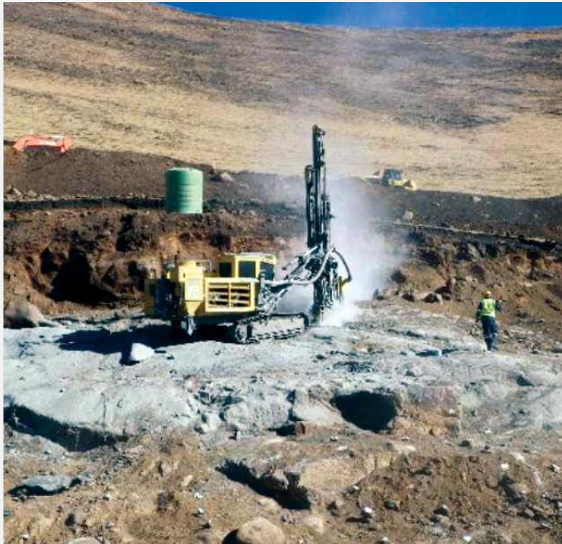
Substation terrace in progress September 2014
