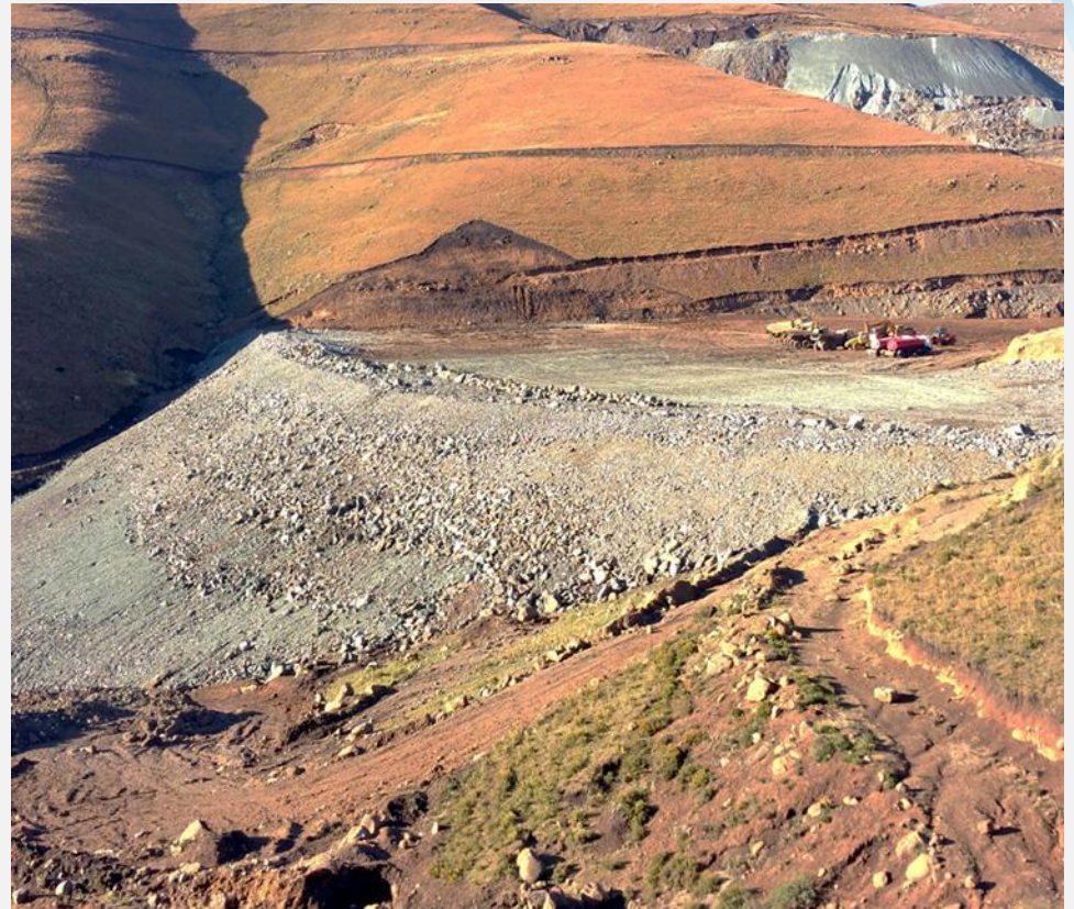
Toe of new slimes dam wall May 2015
