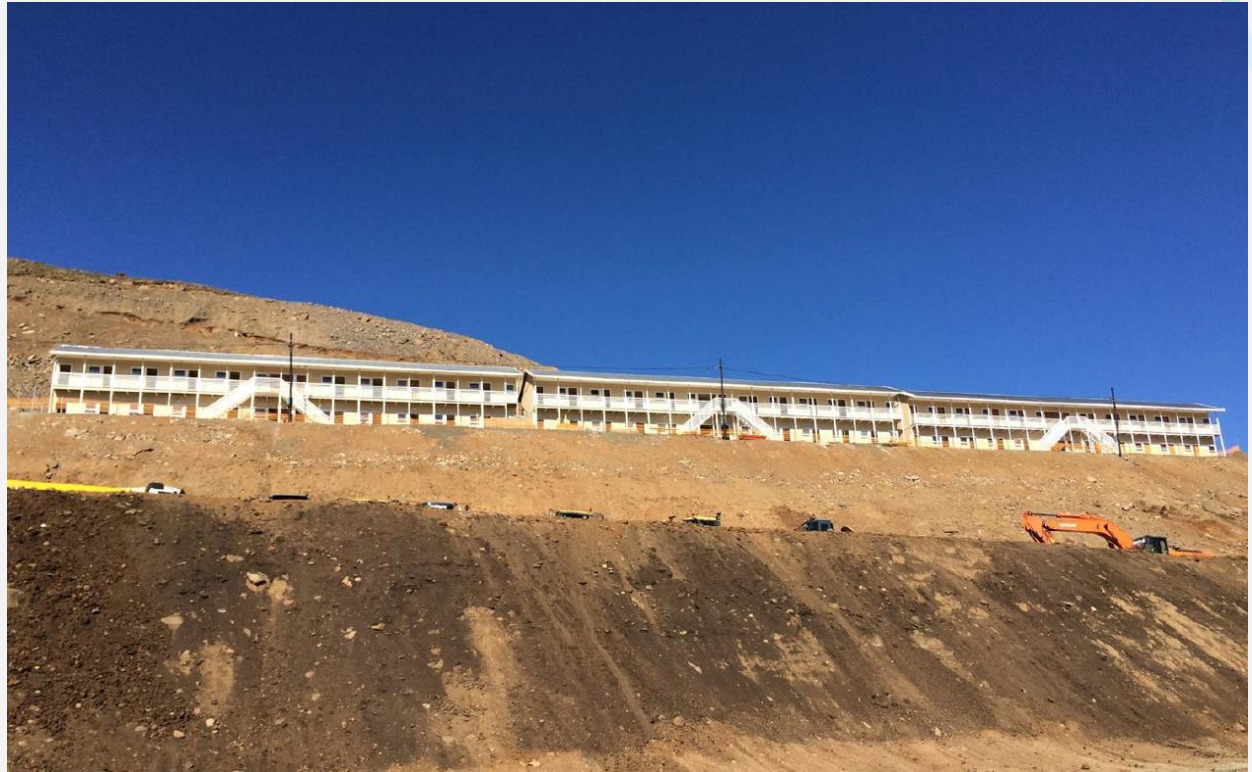
First 3 accommodation blocks ready for occupation May 2015
